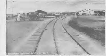
HIRD RAIL was installed in earliest days handle 60-inch standard-gauge flat cars pulled by narrow-gauge locomotives.
